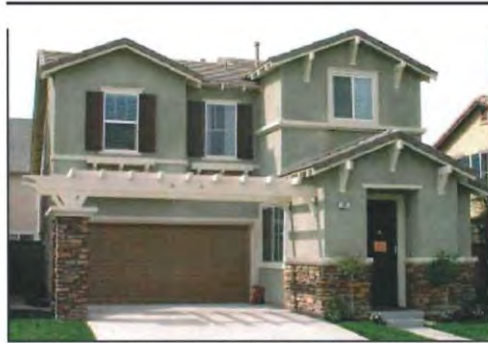
3.3.3 6 a) Recessed garages give importance to the entry and create a pedestrian friendly neighborhood.
